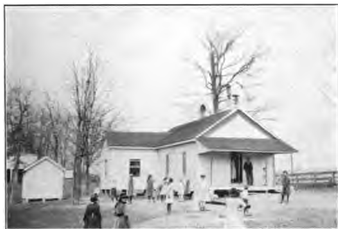
Two- and Three-Room Rural Schoolhouses of the Older Type
